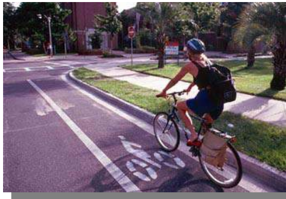
Figure 4.1 Marked Bike Lane Source: www.pedbikeimages.com
