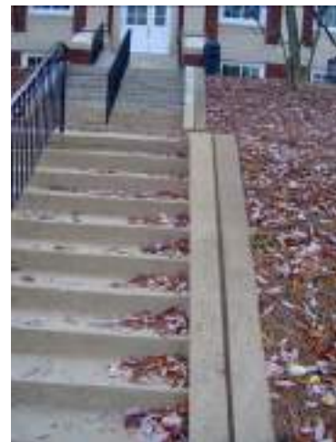
Figure 4.18. Stair channel (Brown Building photo).
