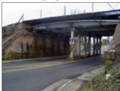
Figure 3.10. Tate Street underpass
