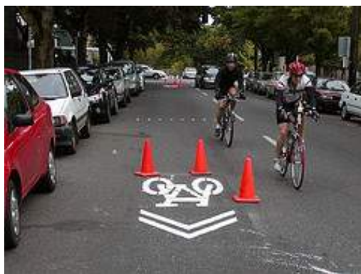
Figure 4.10. Newly-painted sharrow facility in Portland, OR. Source: Todd Boulanger, www.bikeportland.org
